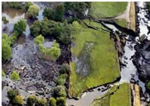
Levee breakthrough (drought)
