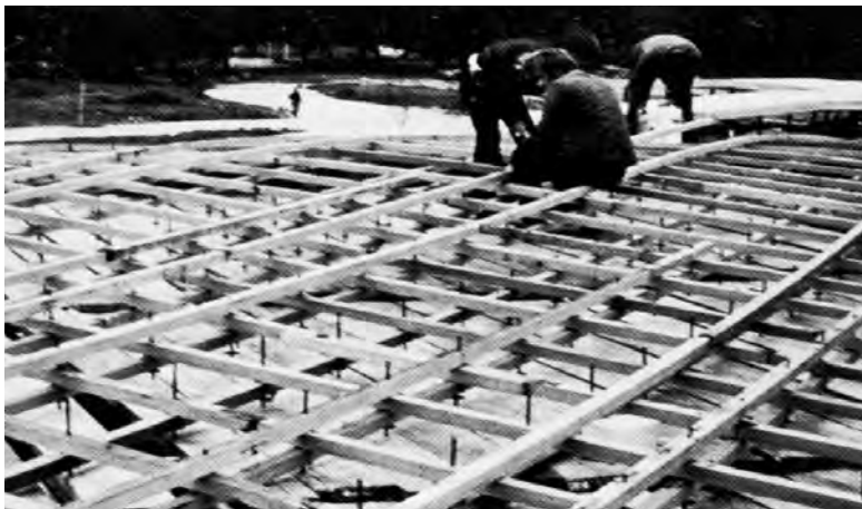
MULTIHALLE MANNHEIM, erecting process from the ground
