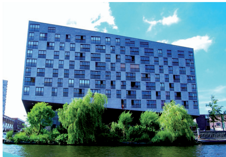
Floating garden in front of an apartment building, in winter and summer Sporenburg, Amsterdam
