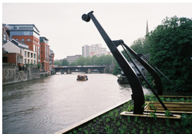
The floating garden uses a smart irrigation system that circulates water from the canal; the lighting is powered by solar panels
