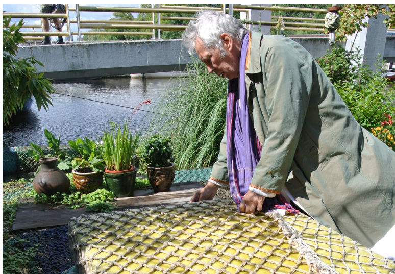
Arie Taal explains how to build a floating garden with EPS and rope
