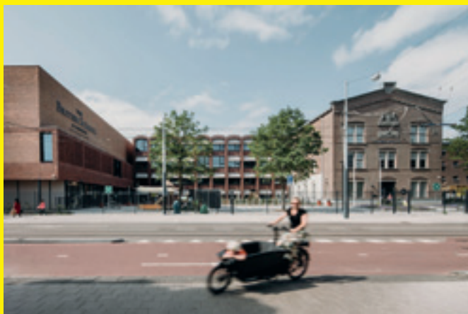
> The British School of Amsterdam Architect: Atelier PRO architecten Opdrachtgever: The British School of Amsterdam Bouwperiode: 2018-09-28 tot 2021-01-06 Fotograaf: Eva Blom
