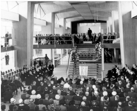
Origineel interieur, centrale hal - 1963
